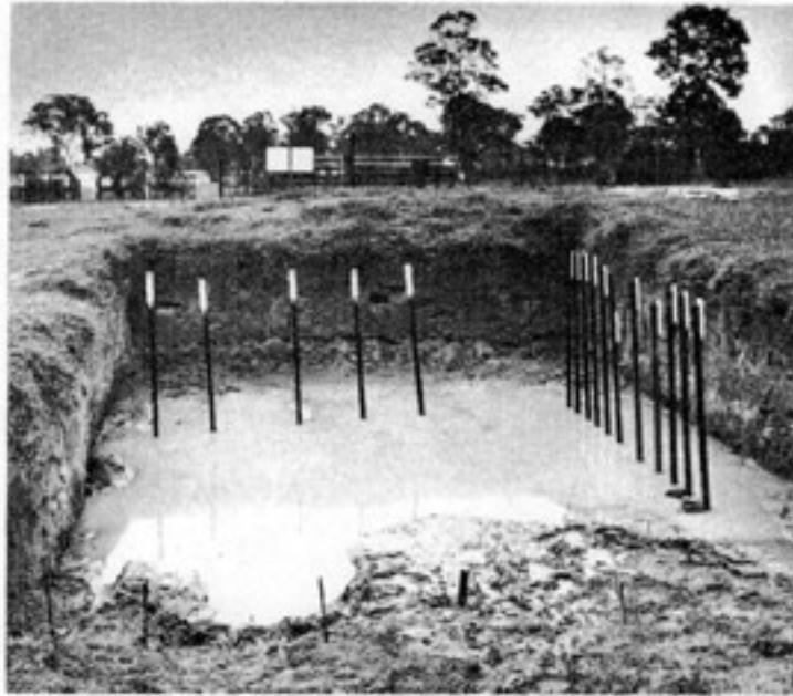
Flooded tank scrape
